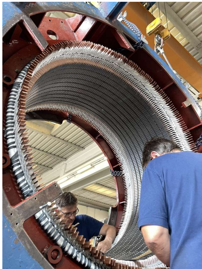
Figure 6: Overhaul and rewinding of a Marelli generator for a hydroelectric power plant, 22,000 Nm.
