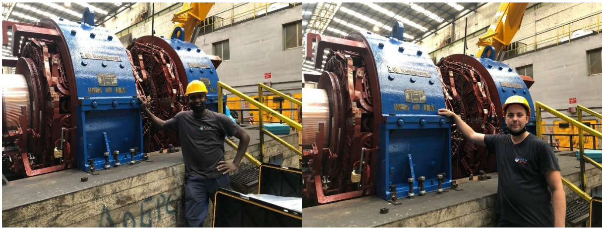
Figures 27 - 28: On-site service, overhaul and installation.
